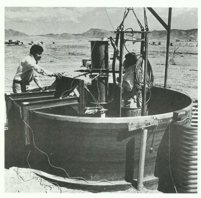
VERTICAL SHOCK TUBE in Coyote Test Field is readied for a test of space RTG units. Manny Vigil and Tom Witherspoon (both 9335) install instrumentation. Tube is 6 metres long; 7½ kilograms of HE was detonated at the bottom of pipe to simulate a launch pad explosion.
